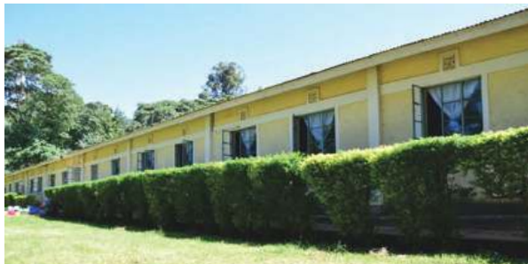
Boarding Facilities at Lugulu Primary School
